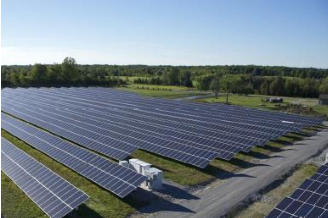
Image 4.2 Option B - Typical Single Axis Trackers
