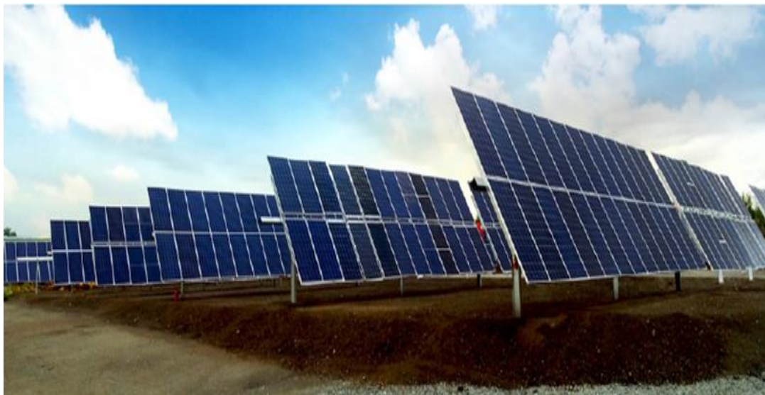
Image 4.2 Option B - Typical Single Axis Trackers
