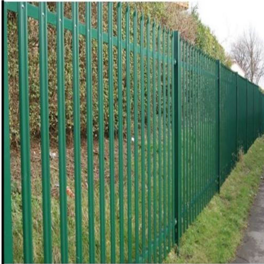
Image 5.8 Typical Palisade fencing
