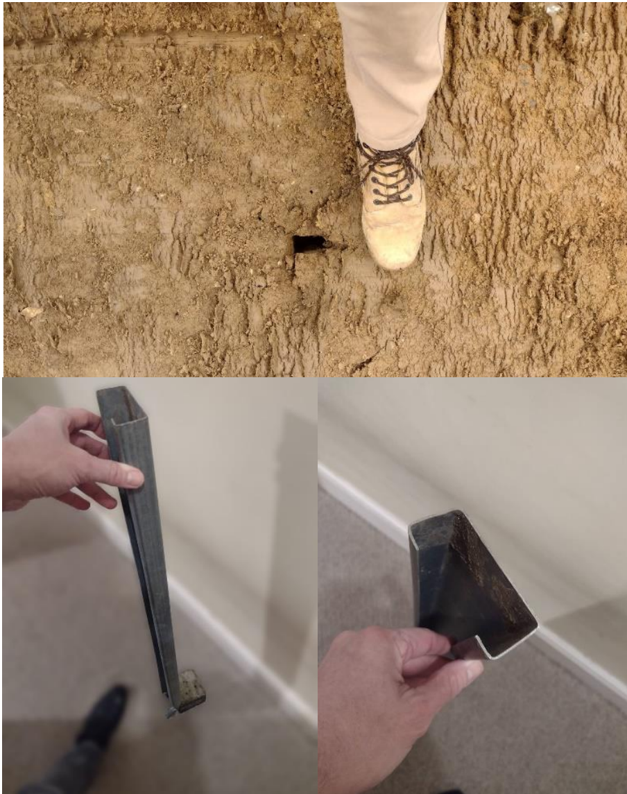
Image 12.4 Typical PV Mounting System pile and physical footprint 3
